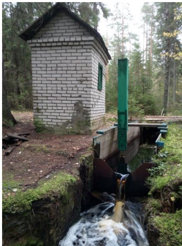
Figure 9. The thin-walled triangular (V-notch) weir on the Zapadnyi stream 1.
